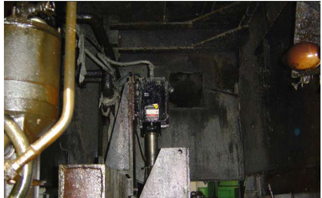
Exit of Cold Rolling Mill
